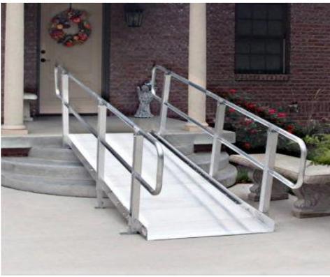
*Pictured above is a customized ramp, placed over existing stairs, that accommodates a motorized wheelchair. Retrieved from: <https://101mobility.com>*
